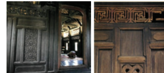
Figure 27: (i) Masjid Telok Manok, Thailand (Noor, F., & Khoo, E., 2013) (ii) Masjid Telok Manok, Thailand (Noor, F., & Khoo, E., 2013)
