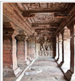
Figure 66: Swastika on the ceiling of Badami Temple (Channappa, 2012)
